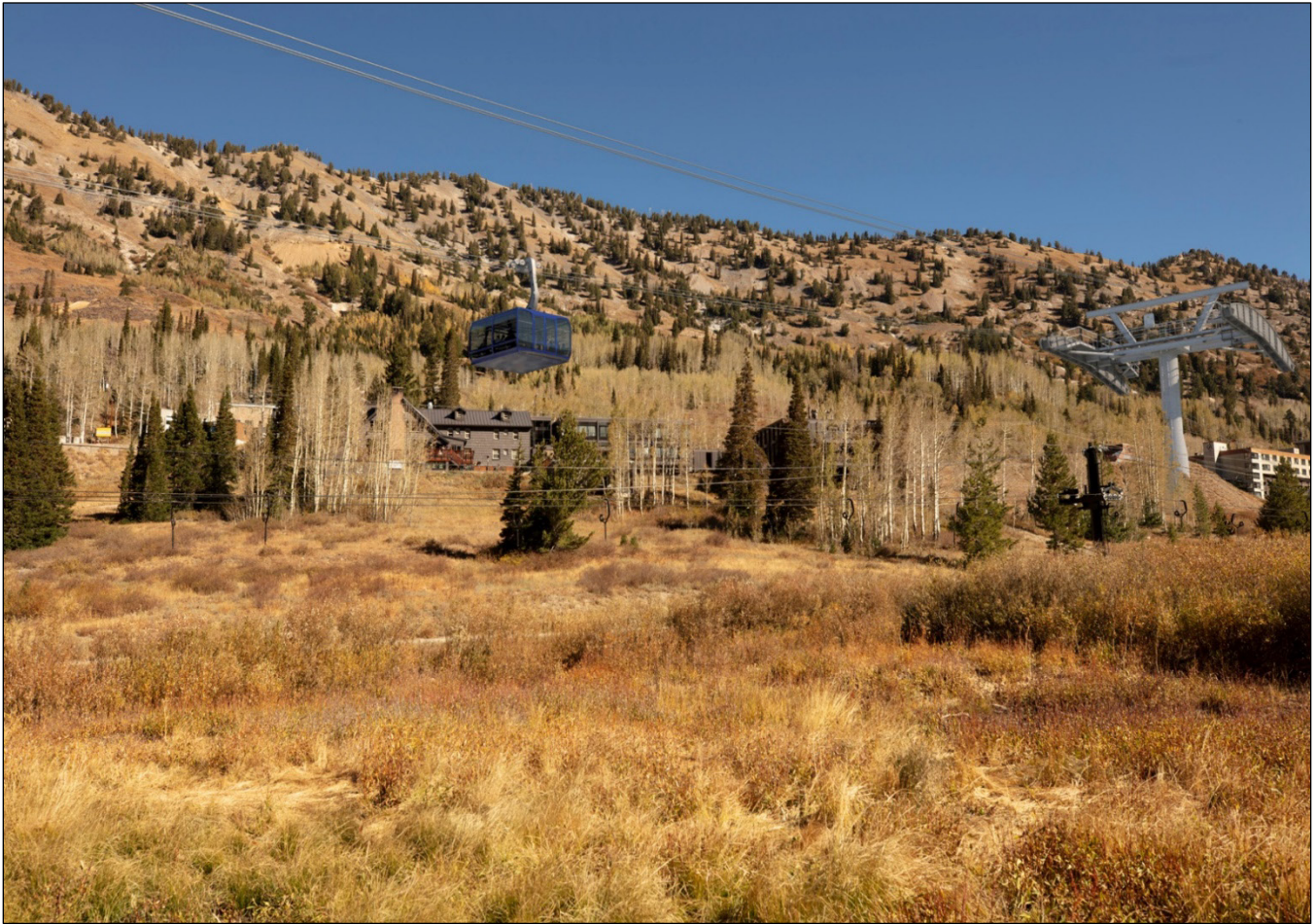
Figure 32E.2-4. Simulated View toward S.R. 210 – Monopole Tower
