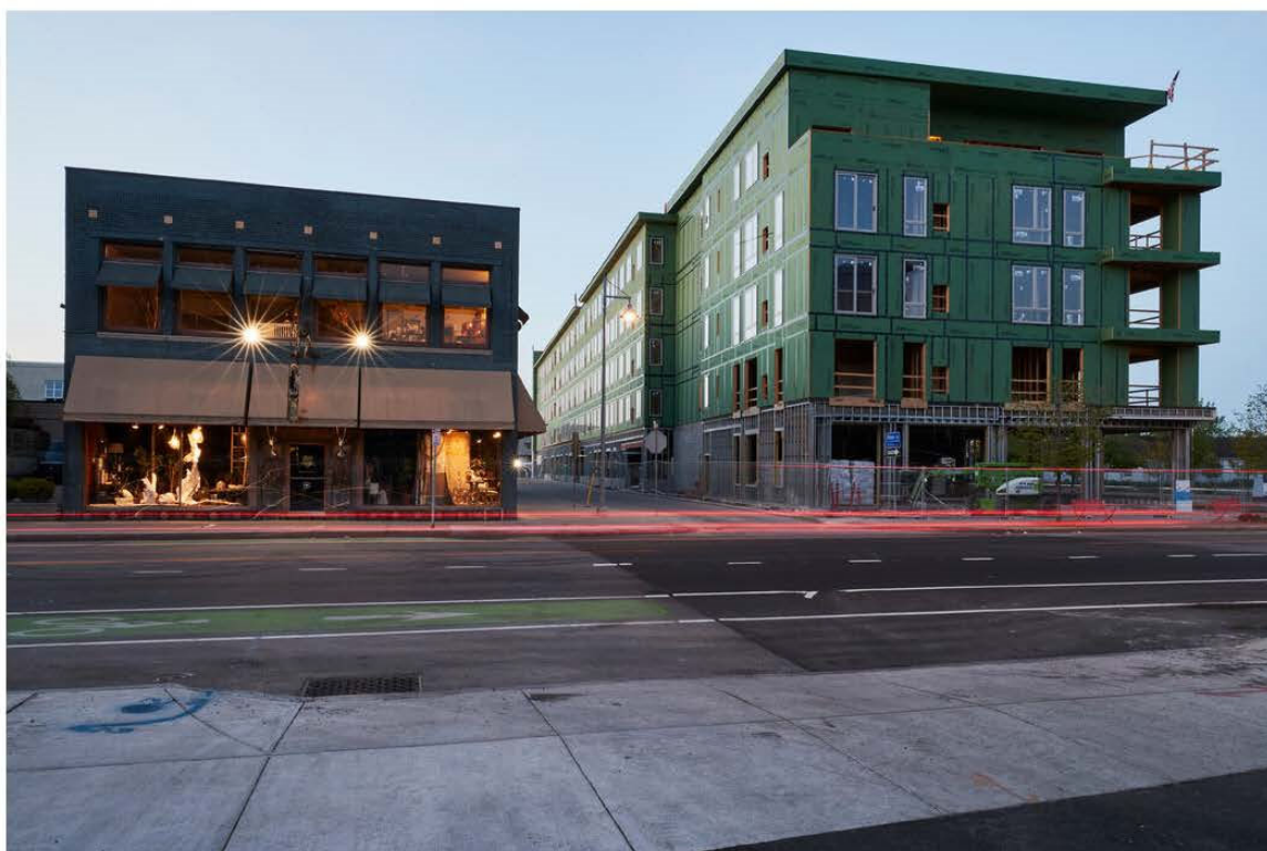
A new apartment building under construction, next to a florist and interior design shop that sat atop the highway for decades. Mustafa Hussain for The New York Times
