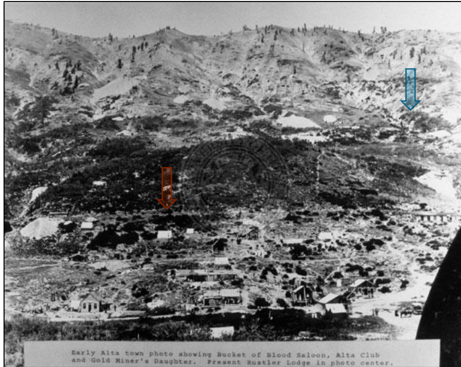
Early Alta town photo showing Bucket of Blood Saloon, Alta Club and Gold Miner's Daughter. Present Rustler Lodge in photo center. Figure A-4. Photograph from the 1890s or early twentieth century showing the beginnings of the Tom Moore Dump (red arrow). The upper workings of the Flagstaff Mine are also visible (blue arrow). Image courtesy of Utah Ski Archives Photos, The University of Utah, J. Willard Marriott Digital Library. Available at: https://collections.lib.utah.edu/ark:/87278/s6w95z05 .
