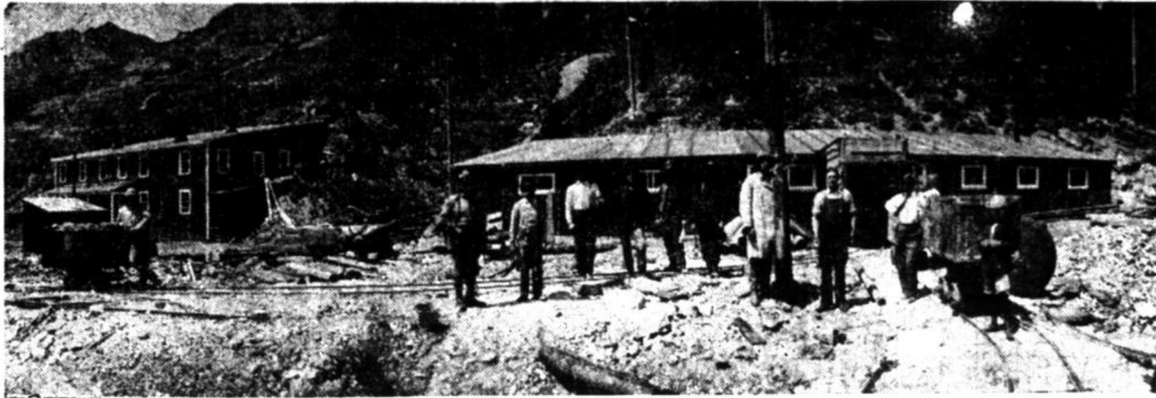
FLAGSTAFF AND EMMA COPPER CO. TUNNEL AND WORKINGS.
