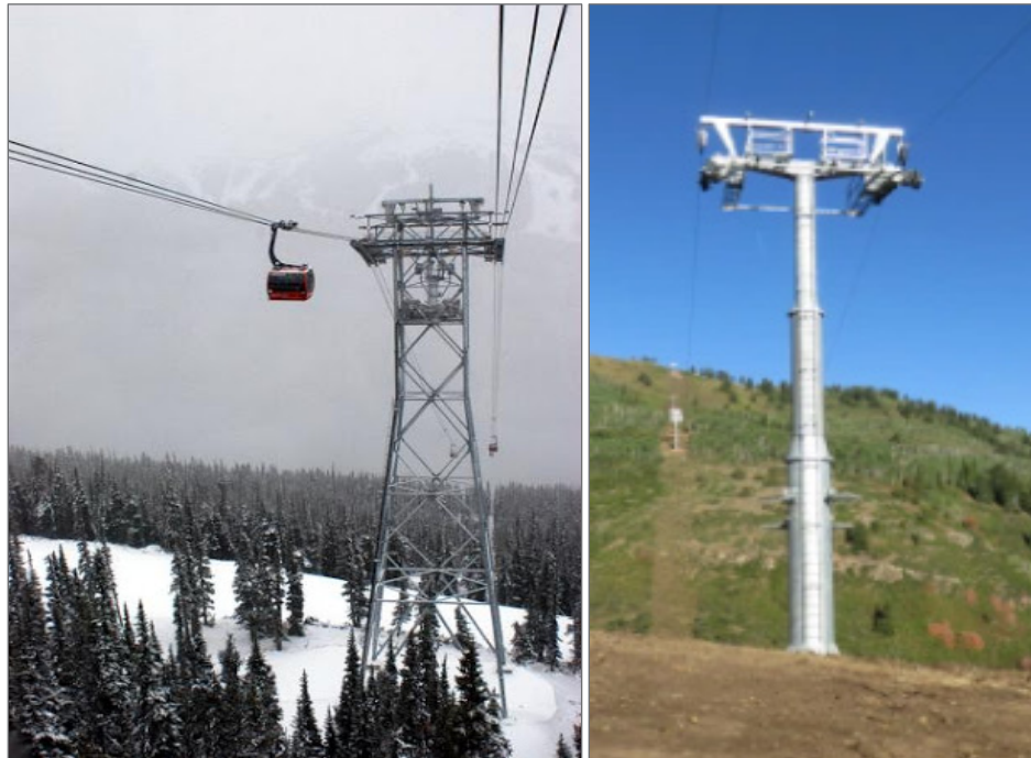
Example lattice tower (left) and pole tower (right).
